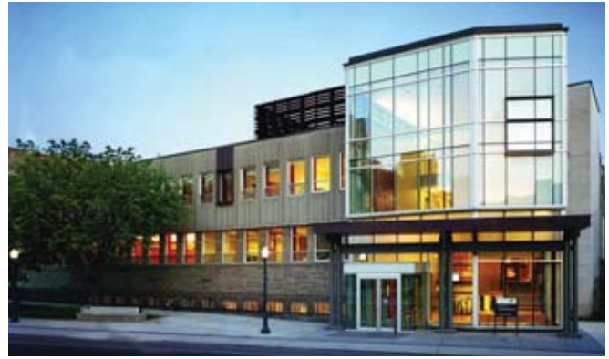
2003 renovations give Queen's Law a hallmark glass atrium entrance.
